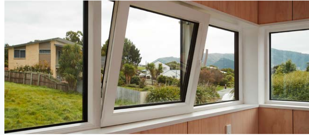
Tilt-and-turn window in hopper mode
